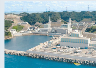
Shimane Nuclear Power Plant
