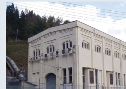
Toyokawa Power Station
