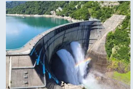
Kamikawa Power Station
